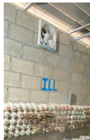
Fig. 8. Location of ventilation fan installation
